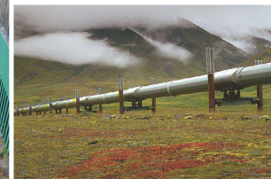
Pipeline 1.2 m diameter Average height 1.5 to 3.0 m
